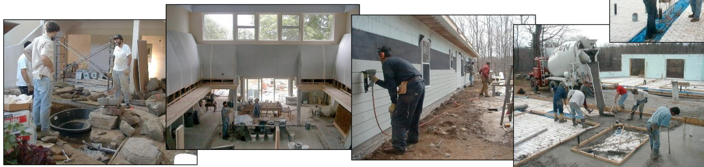
Clockwise: Concrete formwork for exterior walls is halfway up. Starting early morning, in fog, most of the roof trusses go up in a single, long day. Framing of walls and roof. Slab is being prepped. Concrete is being poured for the slab – a major effort. Siding is being installed. The courtyard interior is almost complete. The courtyard fountain and stonework is taking shape.
